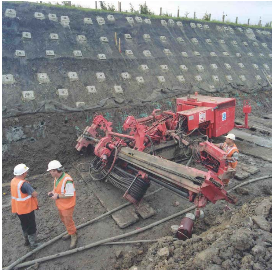
Up to 160 nails are installed every day by six machines
