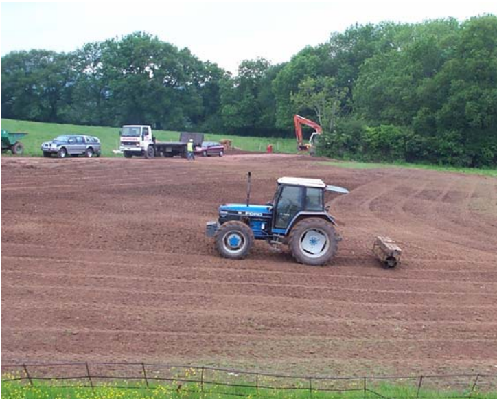
Remediation of Bachy Soletanche working compound
