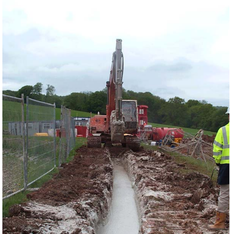
Excavation progressing along dam crest
