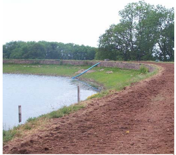
Completed remediation of dam crest
