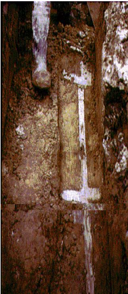
Profile of completed vibwall
