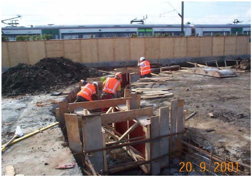
Guide wall construction for piling
