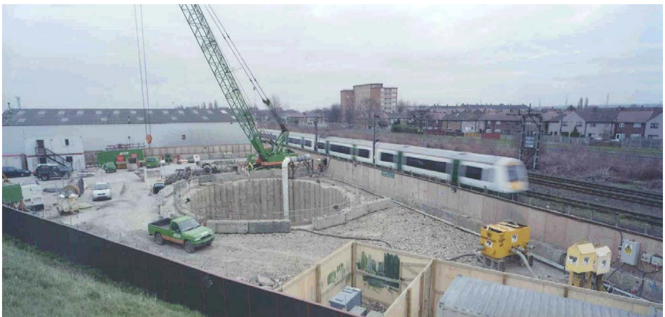
General site view
