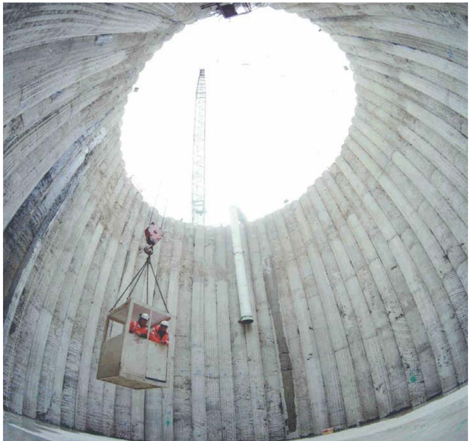
Internal view of shaft from base
