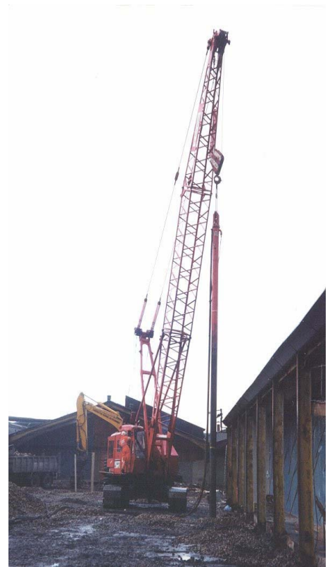
Dry top feed stone columns being constructed at the Tunstall site
