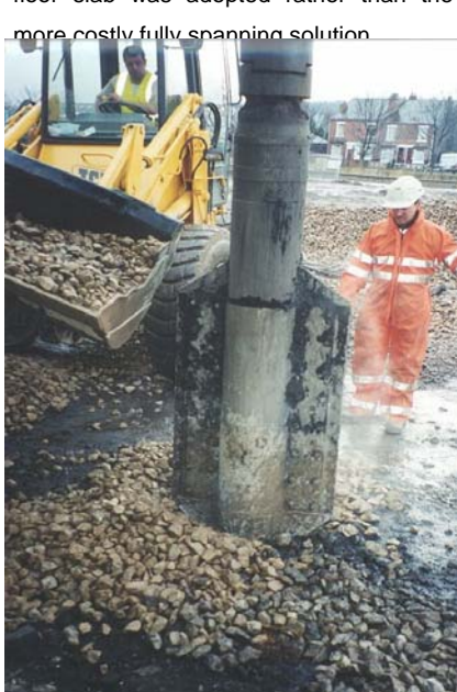
Compaction of Stone into Column
