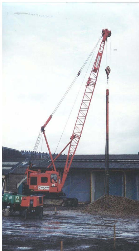
Dry top feed stone columns being constructed at the Tunstall site
