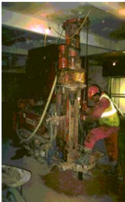
Mini Piling in restricted access areas
