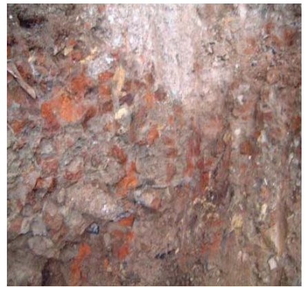
Jet Grouted Wall showing bricks encased in the cement grout matrix
