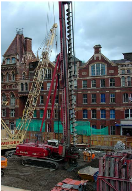
CM700 Rig boring wall piles
