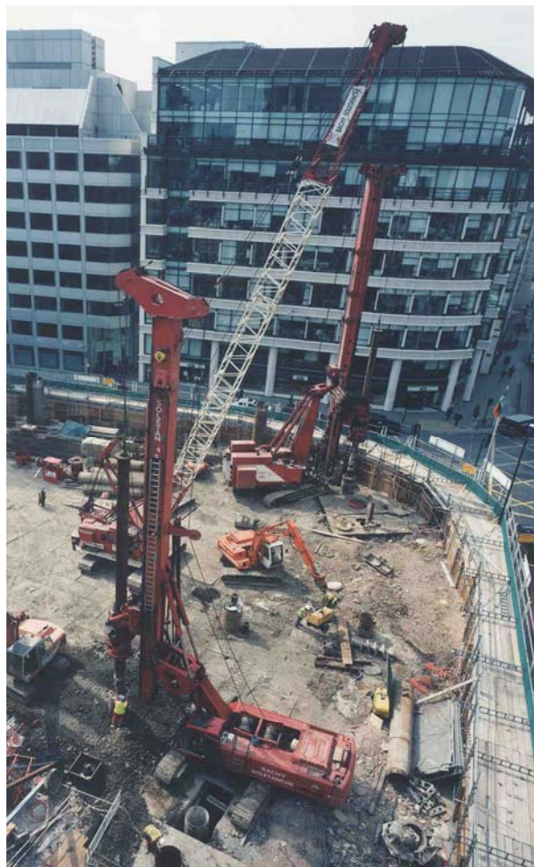
The Construction Site with rigs in place
