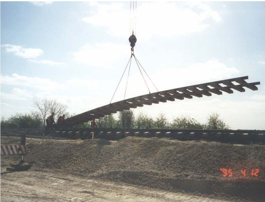
Reinstatement of track onto stabilisation area
