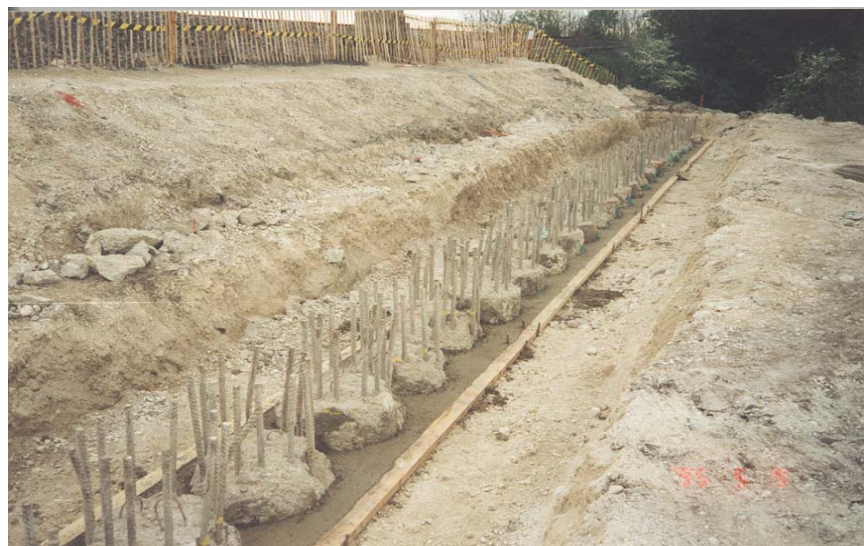
Contiguous bored pile wall construction
