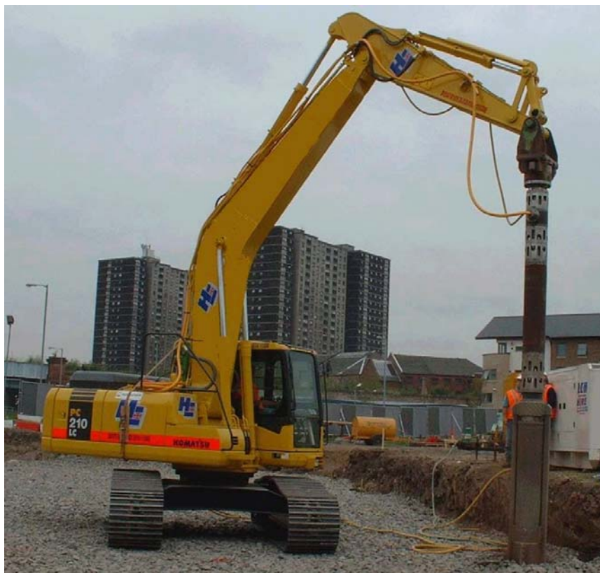
V23 excavator mounted system
