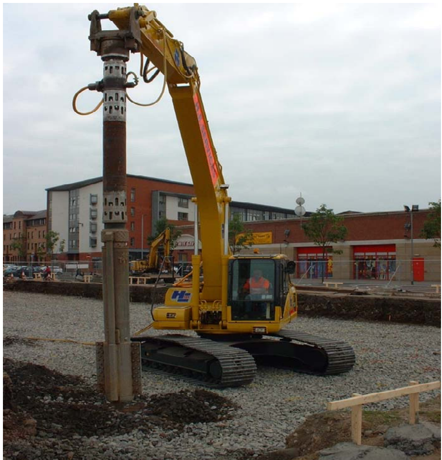
V23 System mounted on a 21 Tonne excavator
