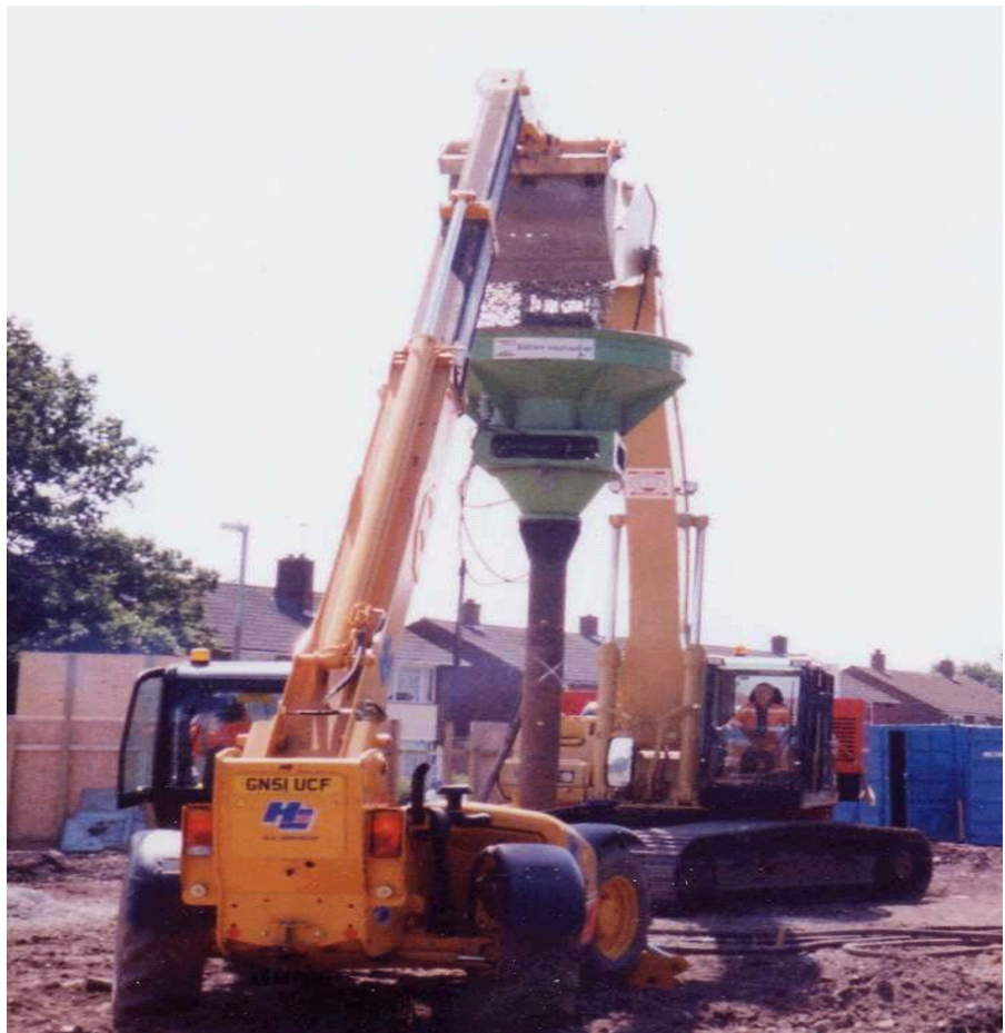
Bottom Feed "Stitcher" System being filled with stone
