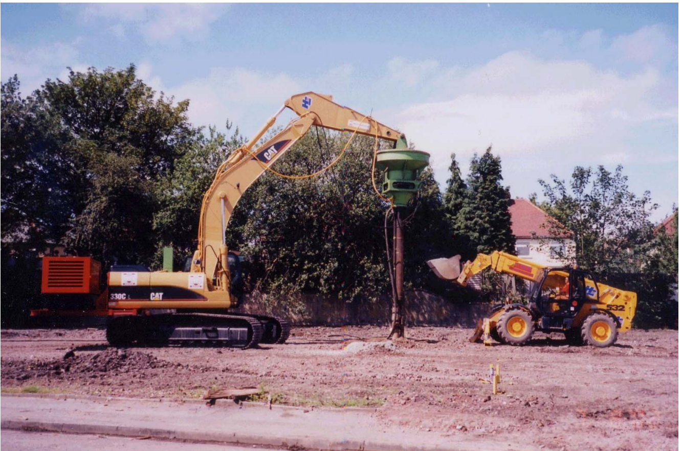
"Stitcher" Assembly constructing a stone column
