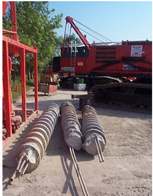
Extracted Screwsol Pile
