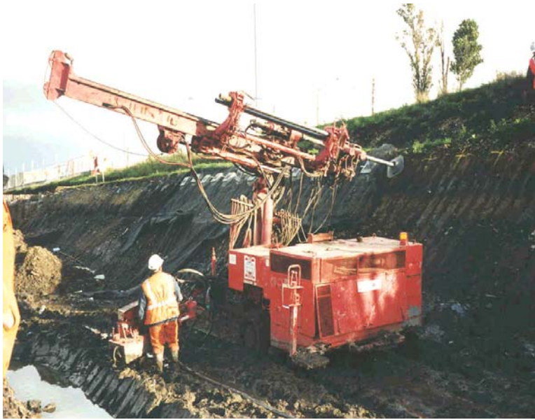
Rig drilling nails 3m above working level using carousel
