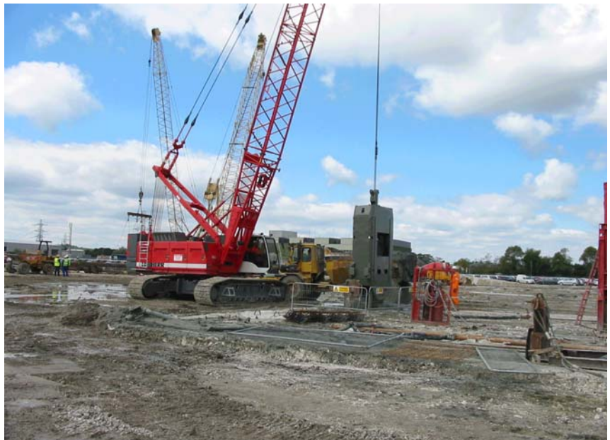
Bunker Structure - Diaphragm Wall construction, grab excavation progress
