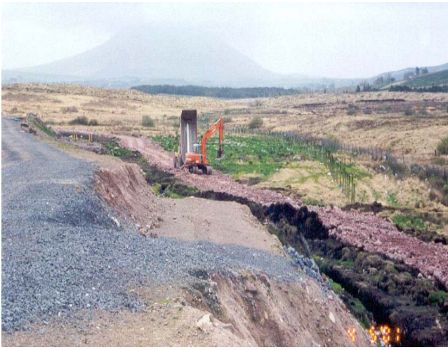
Preparing piling platform
