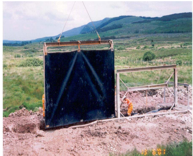
Insertion of HDPE membrane into Slurry Wall
