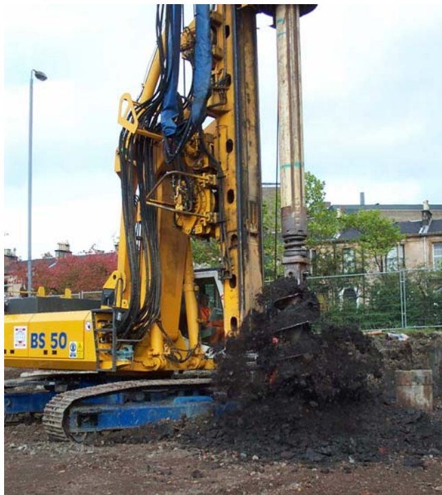
Piling Rig at University of Glasgow
