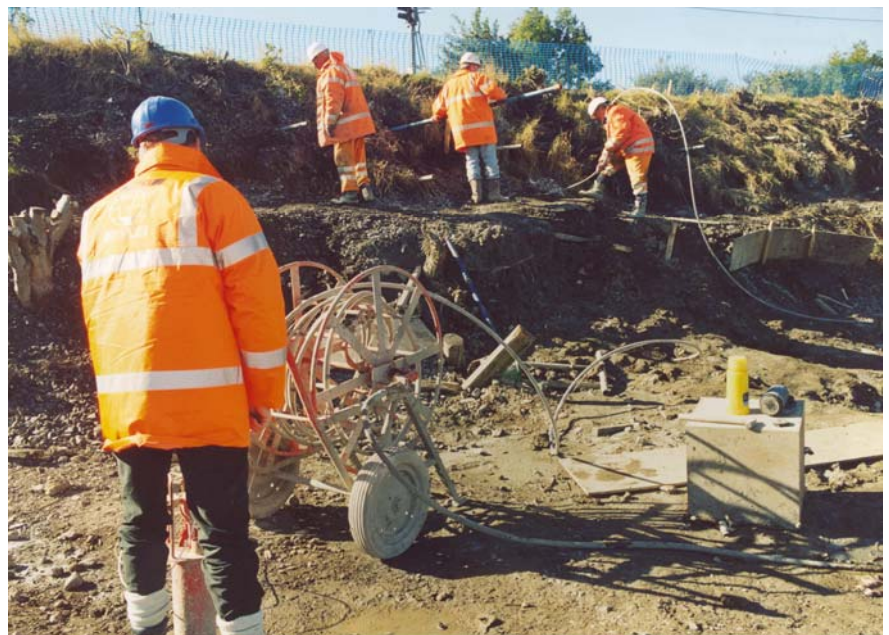
Injection grouters at work
