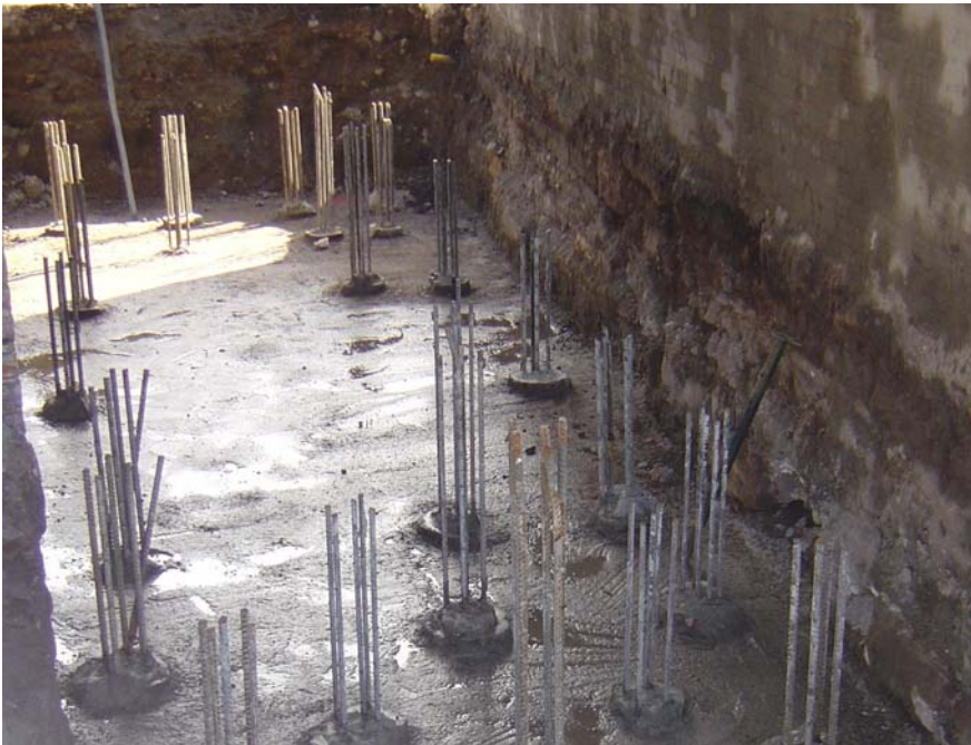
New Viaduct Pier Base
