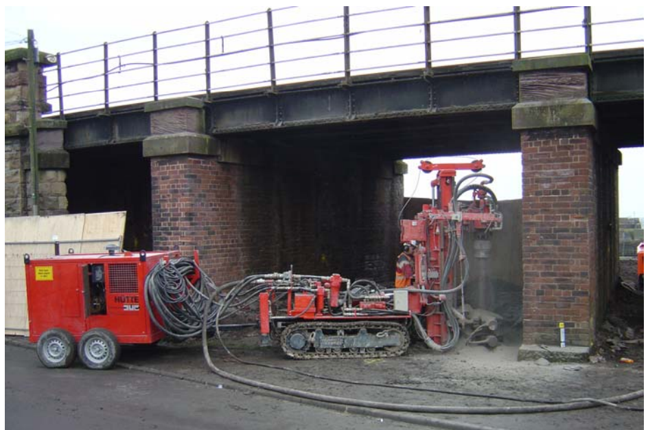
Installing 305mm dia. Mini-piles beneath viaduct
