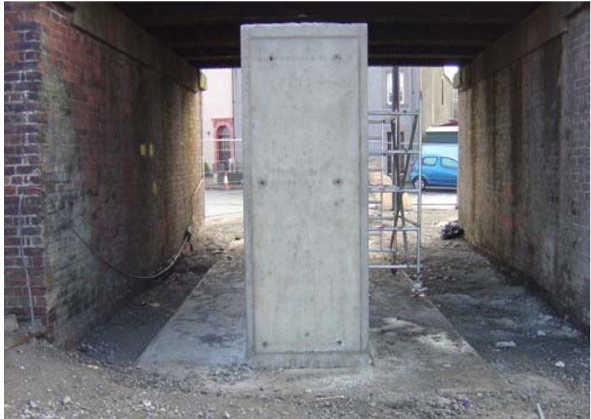
Newly Constructed Viaduct Pier
