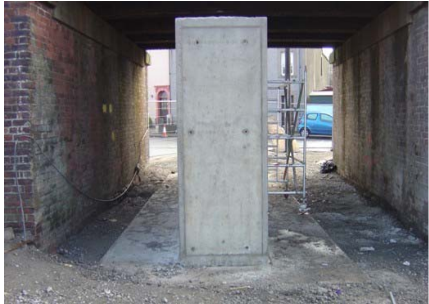
Newly Constructed Viaduct Pier
