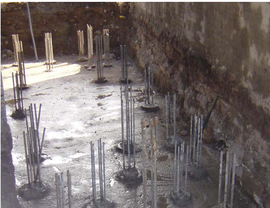
New Viaduct Pier Base
