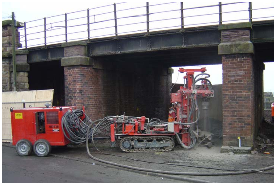
Installing 305mm dia. Mini-piles beneath viaduct
