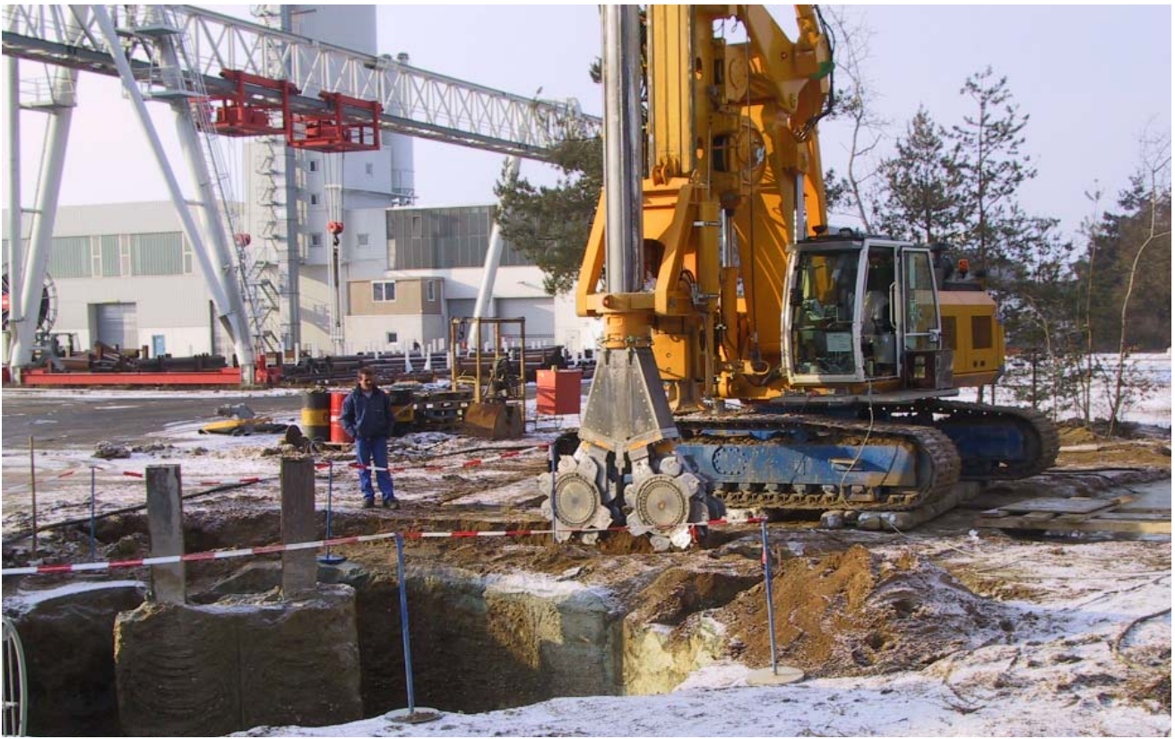
8m diameter CSM shaft
