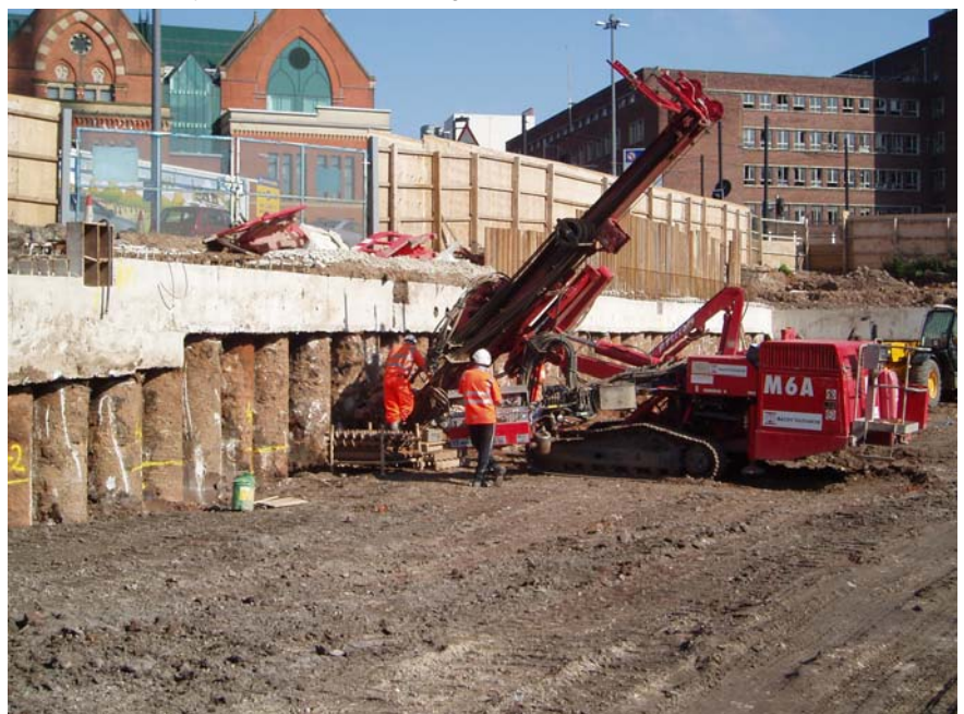
Installation of ground anchors into exposed contiguous piled wall
