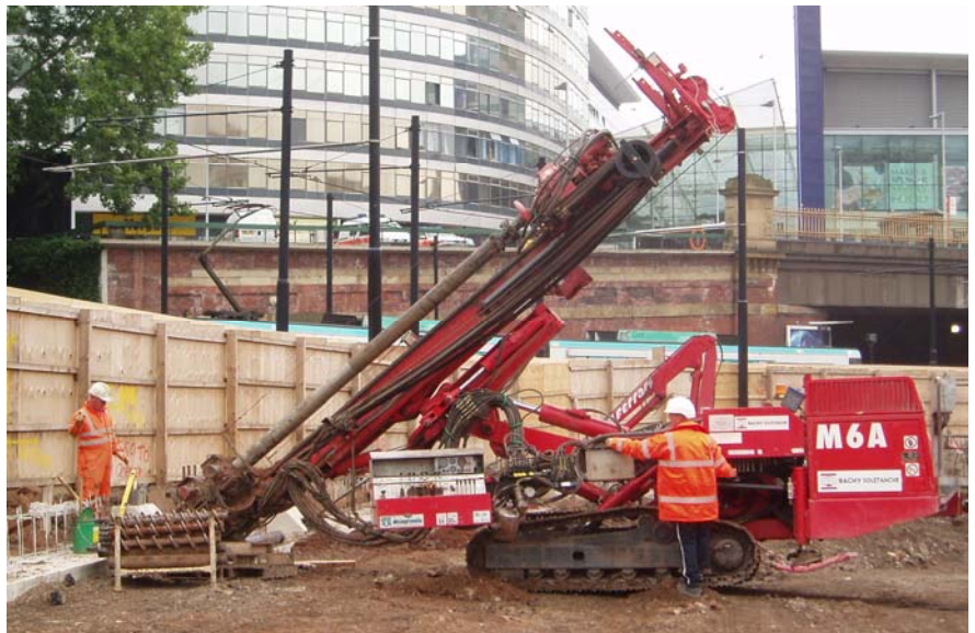
Installation of ground anchors utilising a Casagrande M6 track mounted drill
