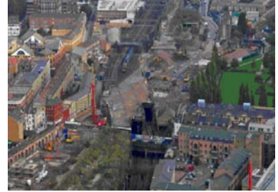
BG30 installing piles for Bridge GE19 just outside Liverpool St Station
