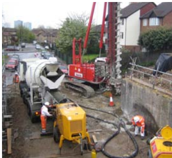
Cold Blow Lane Bridge—CFA piling
