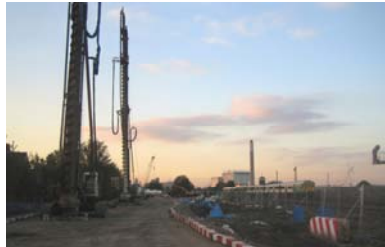
New Cross Gate—Preparing to commence work during a rail possession
