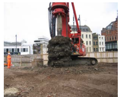
Shoreditch High Street—Large diameter rotary piling, 1500mm diameter.
