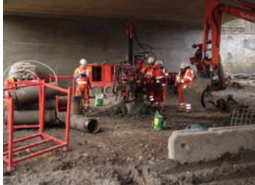
Forest Rd Bridge Restricted Access Mini-piles
