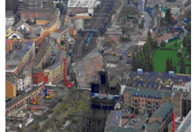
BG30 installing piles for Bridge GE19 just outside Liverpool St Station
