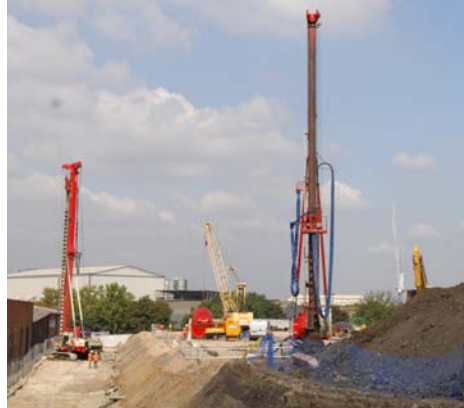
Clockwise from top left: Artist's Impression of the London Overground Rolling Stock, extract from TfL Tube Map showing the new East London Line route as part of the London Overground network and CFA rigs installing piles for New Cross Gate Maintenance Facility.
