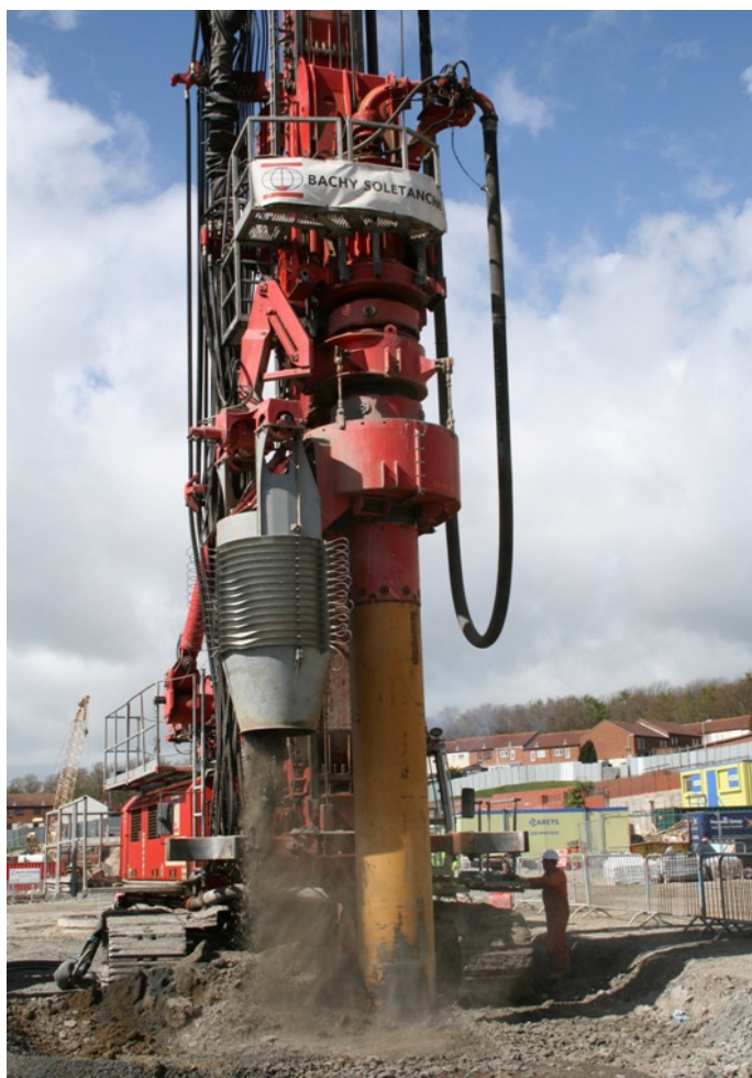
High Torque Cased CFA Rig with soil handler
