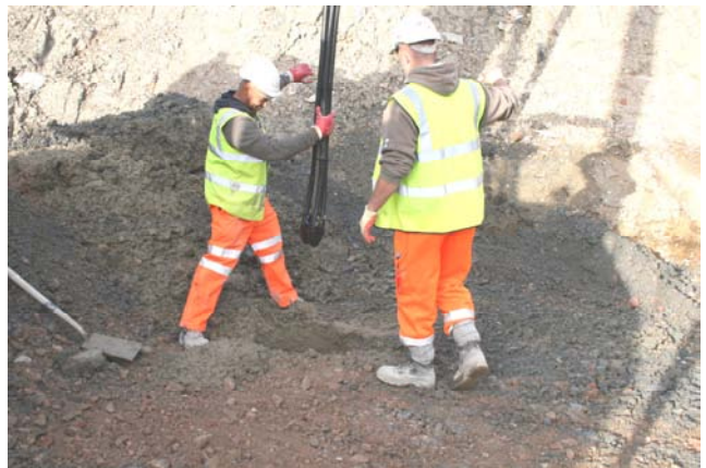
Insertion of Geothermal Piping
