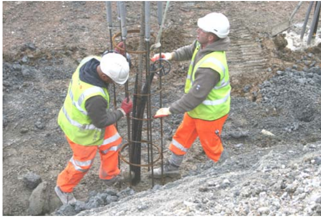
Insertion of piping and reinforcement cage.
