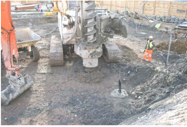
Boring of Pile
