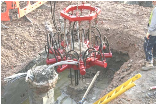
Breaking down of pile after installation
