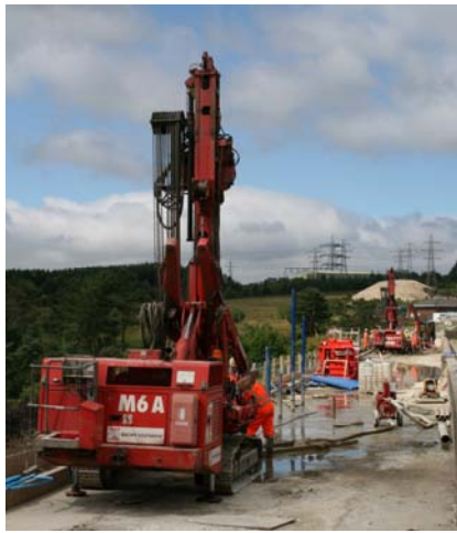
Drilling of grout curtain
