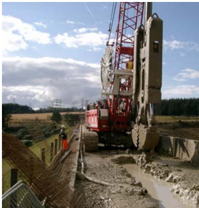
KS Grab digging Cut-off wall
