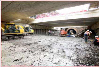
Thameslink Box excavation, also showing the contiguous piled wall
