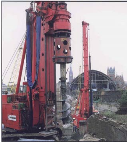
L.D.A. rotary rigs piling the station extension
