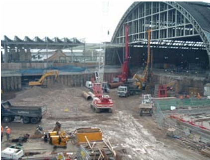
Piling to the west side of the deck extension
