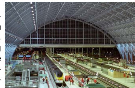
Station just prior to re-opening
