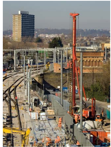
C.F.A. Piling close to live rail
