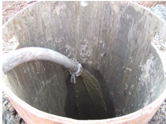
Mixing Plant, Mixed Polymer Solution, and Pumping to Pile
