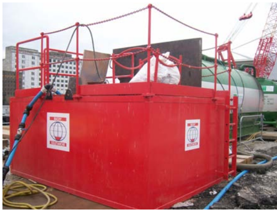
Mixing Plant, Mixed Polymer Solution, and Pumping to Pile
