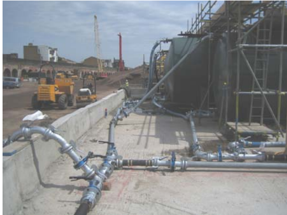
Mixing Plant, Mixed Polymer Solution, and Pumping to Pile
