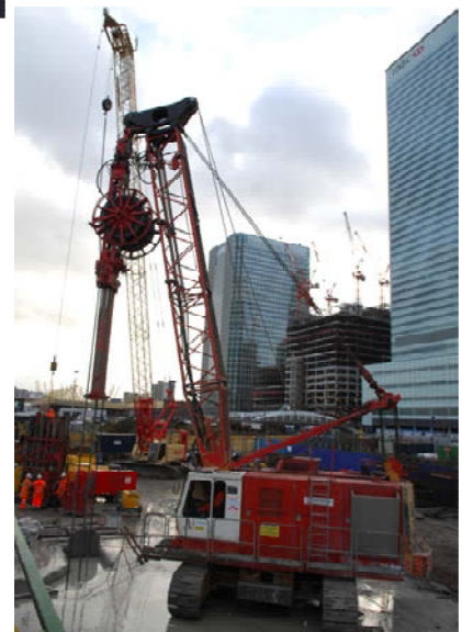
Digging of panel under Bentonite
