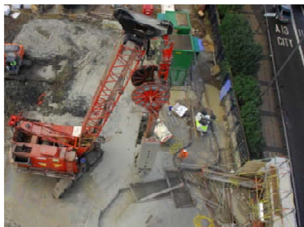
Digging of panel under Bentonite
