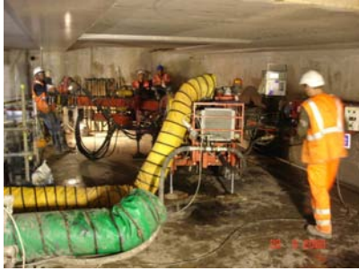
Drilling grouting array
