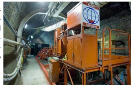
Grout Mixing Equipment
