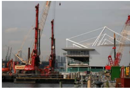
Piling from 2 barges and from the quay
