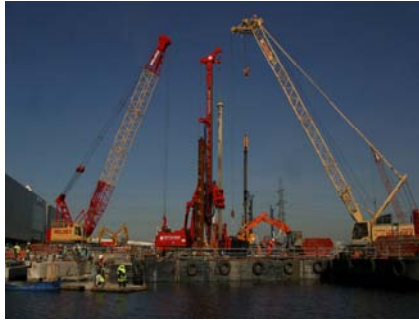
Piling rigs with support cranes
