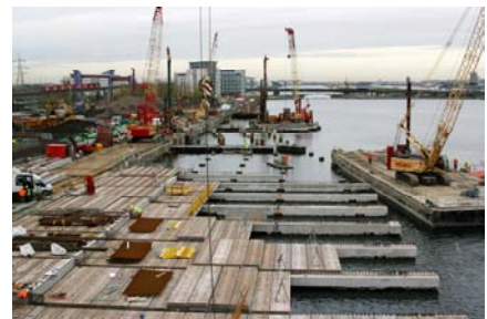
Placing of the precast concrete beams and planks
