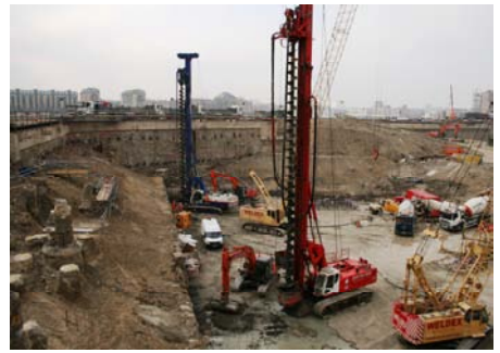
900mm dia. CFA Piling to 27m
