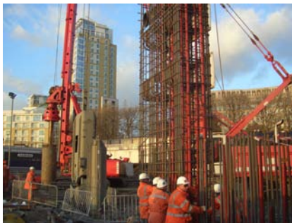
Installation of diaphragm wall cage
