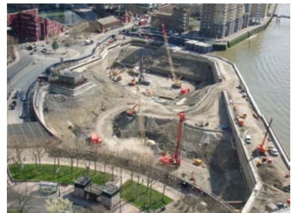
Exposed Diaphragm Wall during excavation and CFA piling
