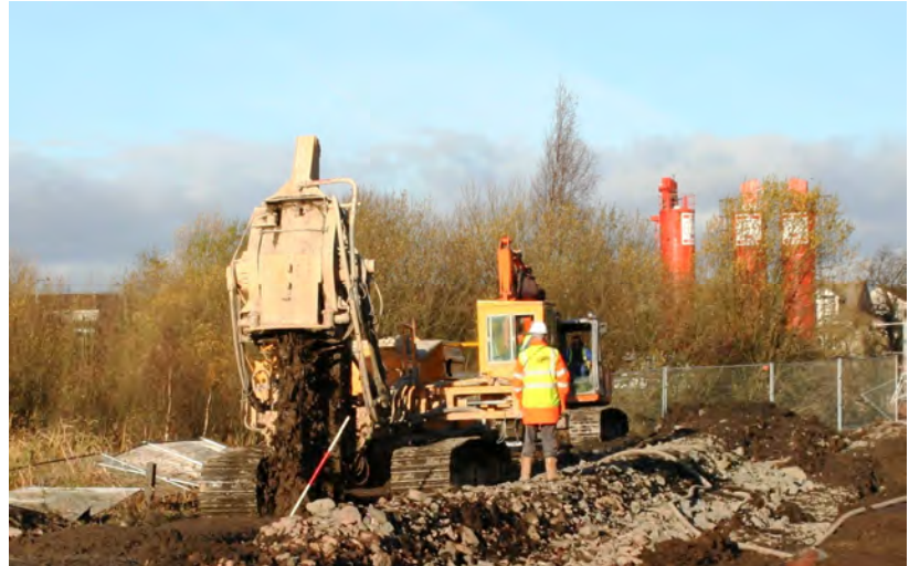
Ground Improvement for a roadway at Steppes, near Glasgow
