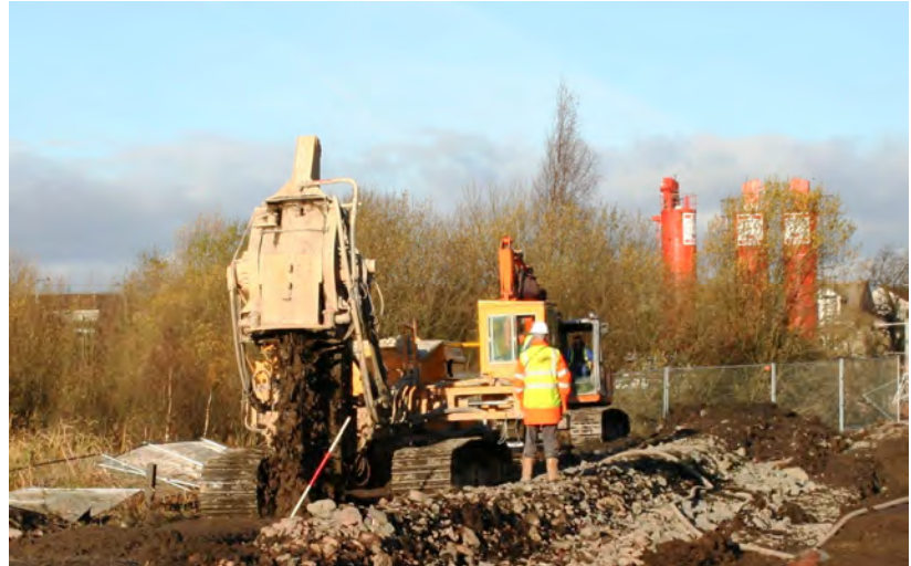
Ground Improvement for a roadway at Steppes, near Glasgow
