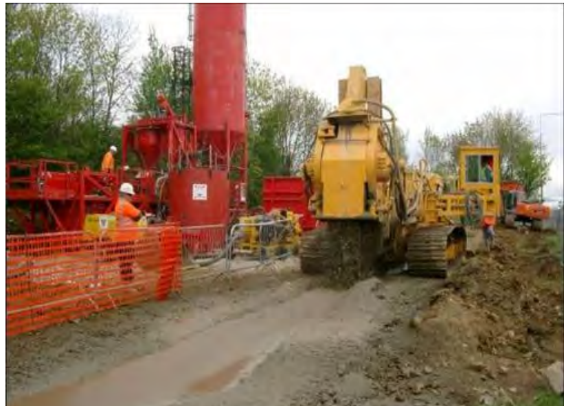
Contamination “Cut-off” Barrier at Bletchley, near Milton Keynes by
