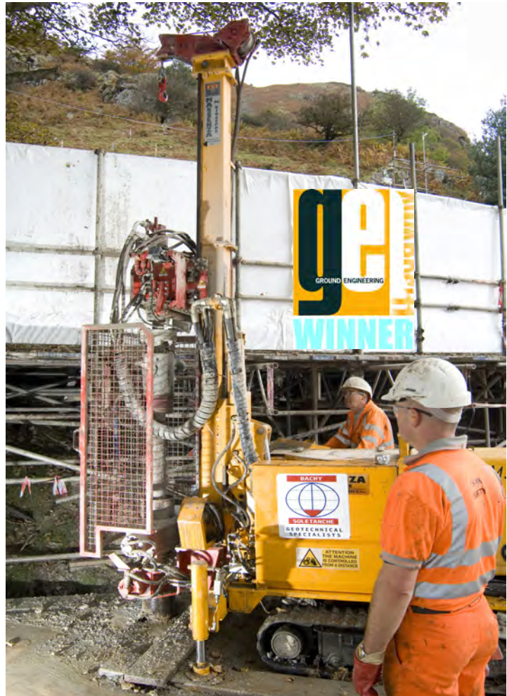
Minipiling on a steep slope
