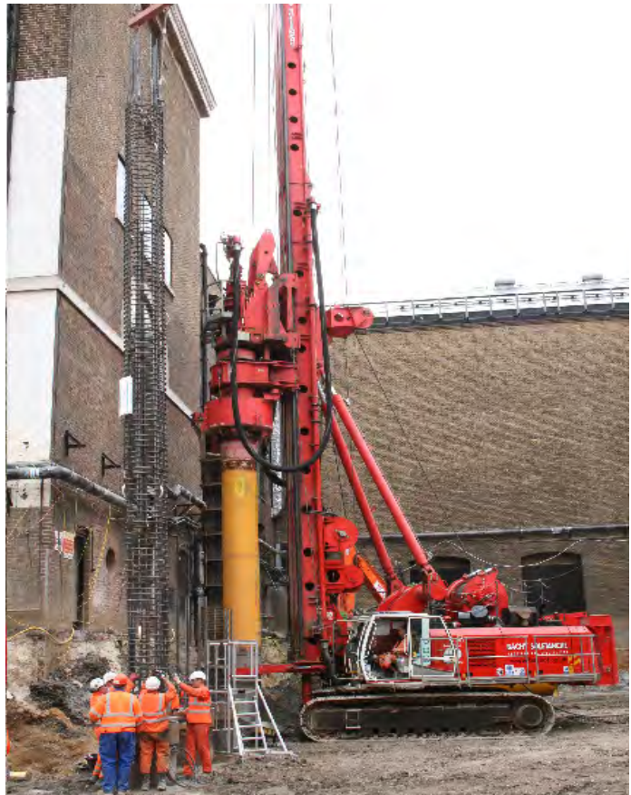
Boring of Cased CFA secant wall pile and cage insertion
