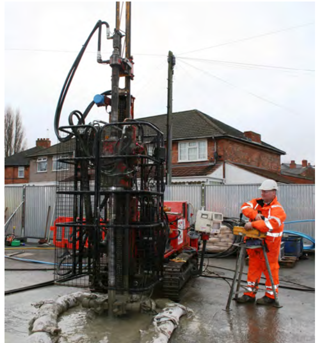
Jet Grouted Column under construction
