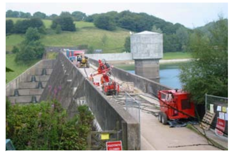
View along crest of dam
