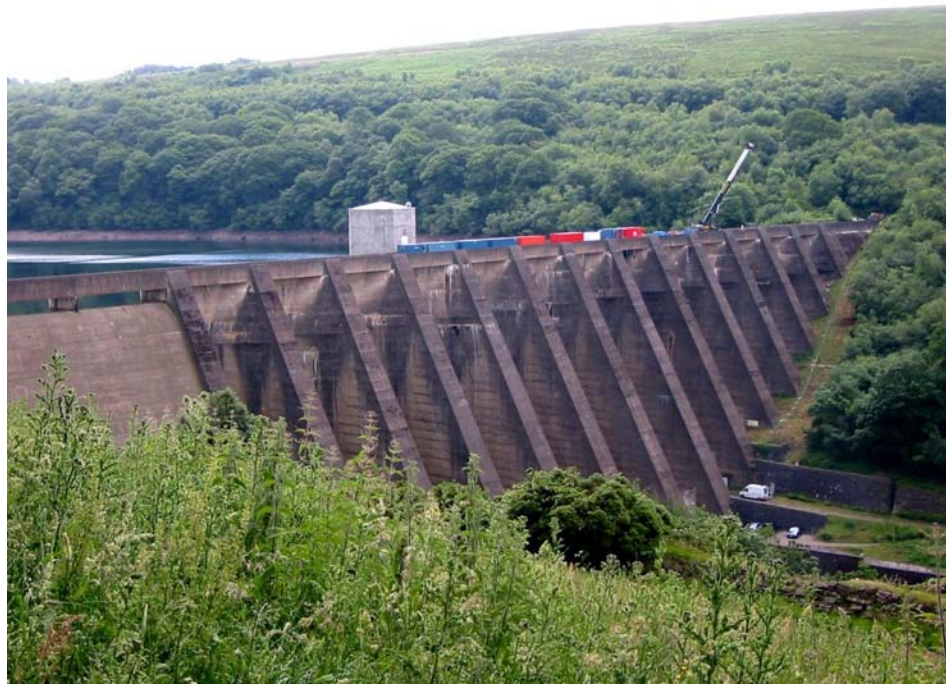
Upstream view of buttresses of Wimbleball Dam
